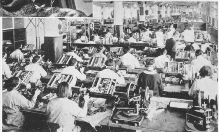
Coils are indispensable in the transmission, control, and protection of telephone currents. These Kearny girls are zinding them on machines.
